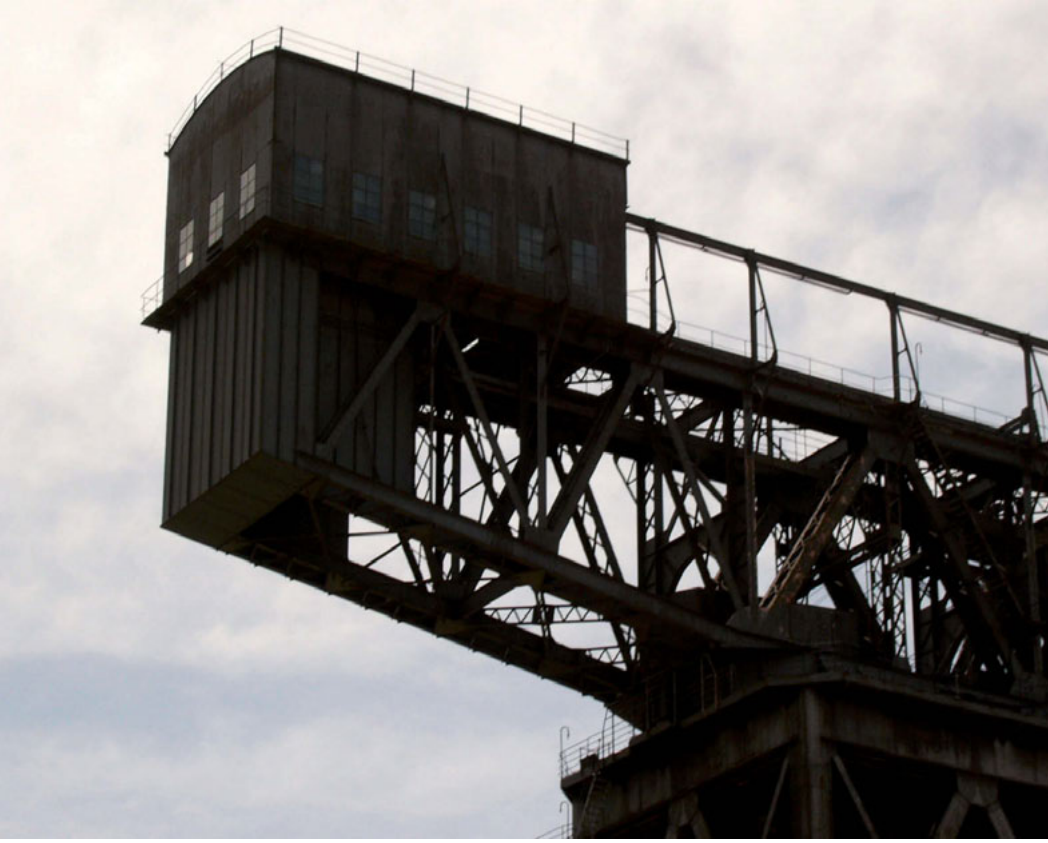
The three illustrations above give a progressive three quarter view of the boom from the engine house to the tip of the boom. There is sufficient detail to enable a builder to reproduce the number of bays and the bracing. Left: Rear cantilever and engine house. Centre: Tower head, turntable and jib centre. Right: Forward boom showing crab and bracing structures. Below right: The traveller and lifting tackle.
