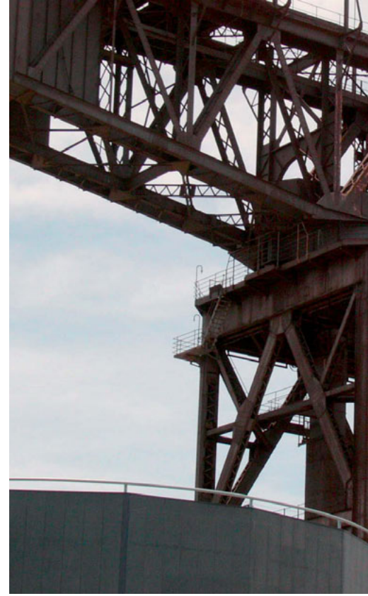
The three illustrations above give a progressive three quarter view of the boom from the engine house to the tip of the boom. There is sufficient detail to enable a builder to reproduce the number of bays and the bracing. Left: Rear cantilever and engine house. Centre: Tower head, turntable and jib centre. Right: Forward boom showing crab and bracing structures. Below right: The traveller and lifting tackle.
